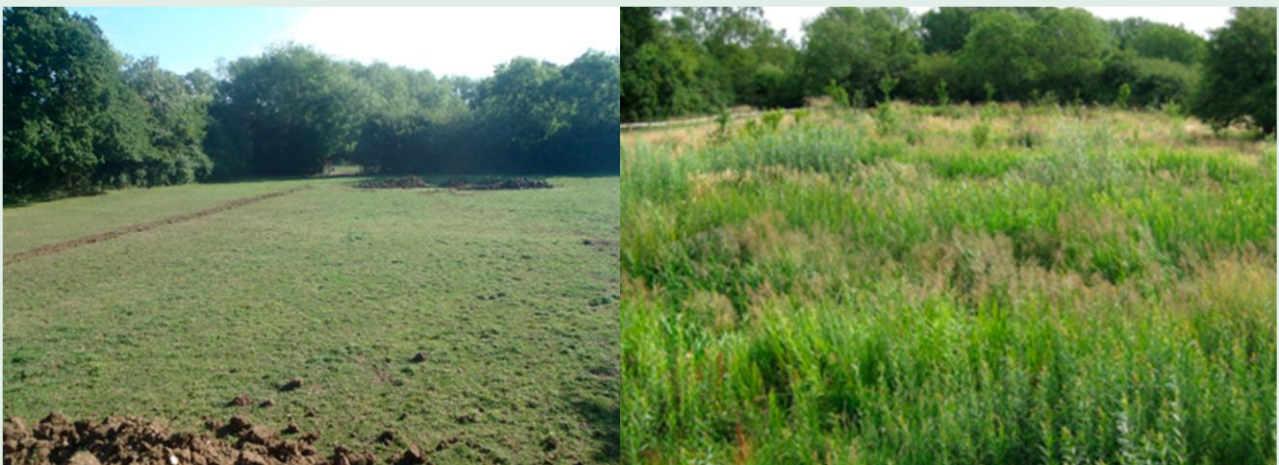
Figure 6: Wastewater treatment area before (compacted horse paddock) and 10 months after, with shrubs and other plants beginning to be established. Photo credit: Jay Abrahams
